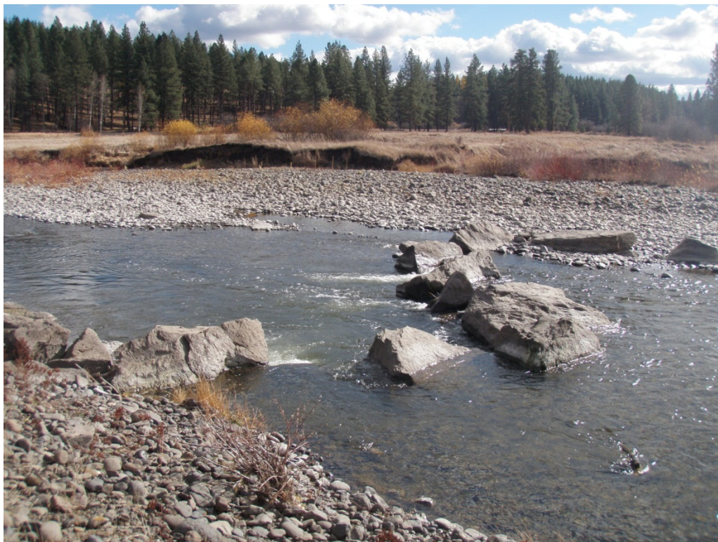
Figure 11. Instream rock structure in the Birdtrack/Longley reach.
